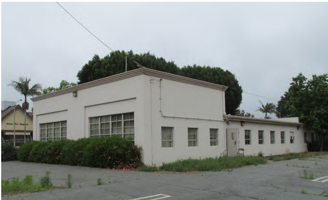
Figure 2. West elevation of Fremont Hall USAR Center, looking northeast. (IMG_8413)
