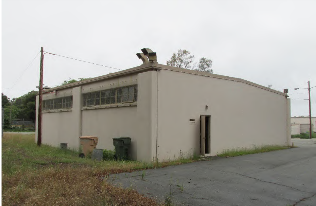
Figure 14. Organizational Maintenance Shop north and east elevations, looking southwest. (IMG_8341)
