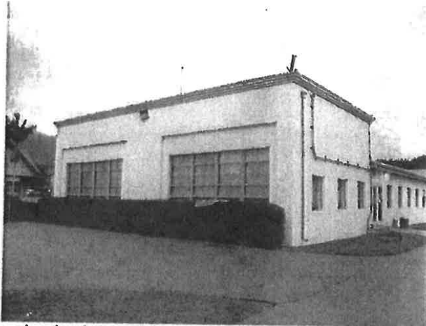
East façade and portion of south façade of center, view northeast, 2-27-06, SBCo-FH-05-5037-026.jpg
